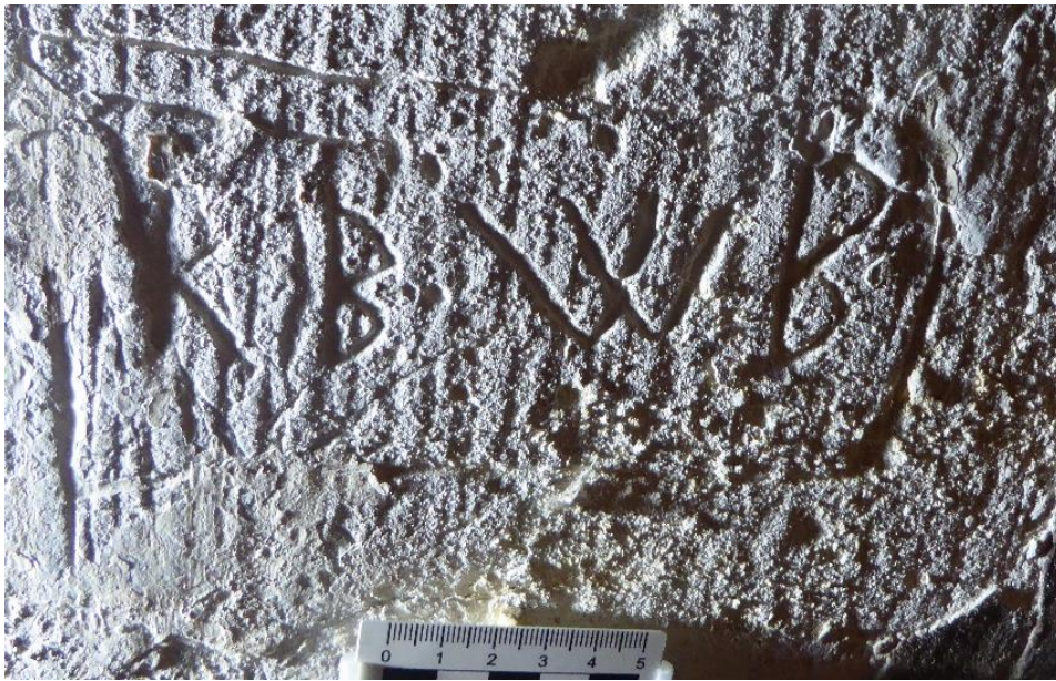
Fig 36. Chancel south doorway. Paired initials RB and WB
