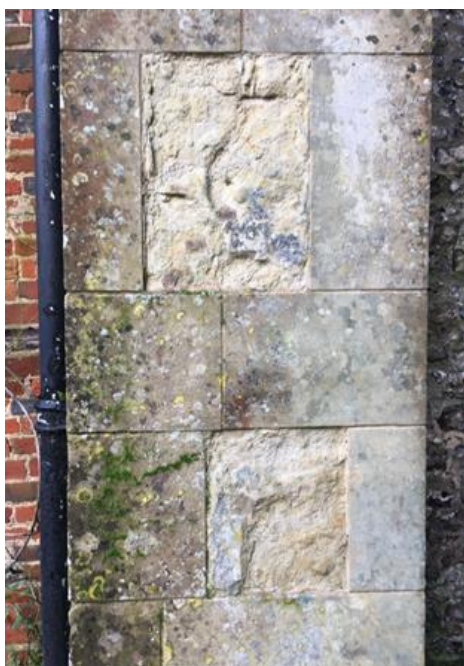
Fig 42 south porch, south buttress. Remains of mass dials
